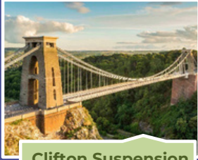
Clifton Suspension Bridge
